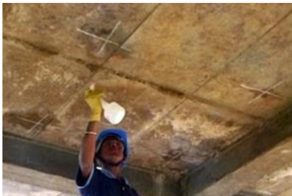
Marking of Slab and Pre-wetting for Half-Cell Potential Test
