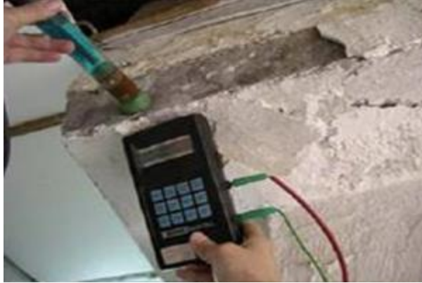
Half-Cell Potential Test of Slab
