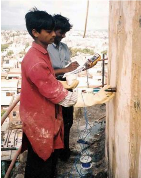
Half-Cell Potential Test of Overhead Water Tank Wall
