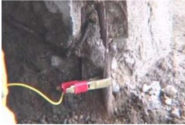
One end of Half-Cell connected to the reinforcement
