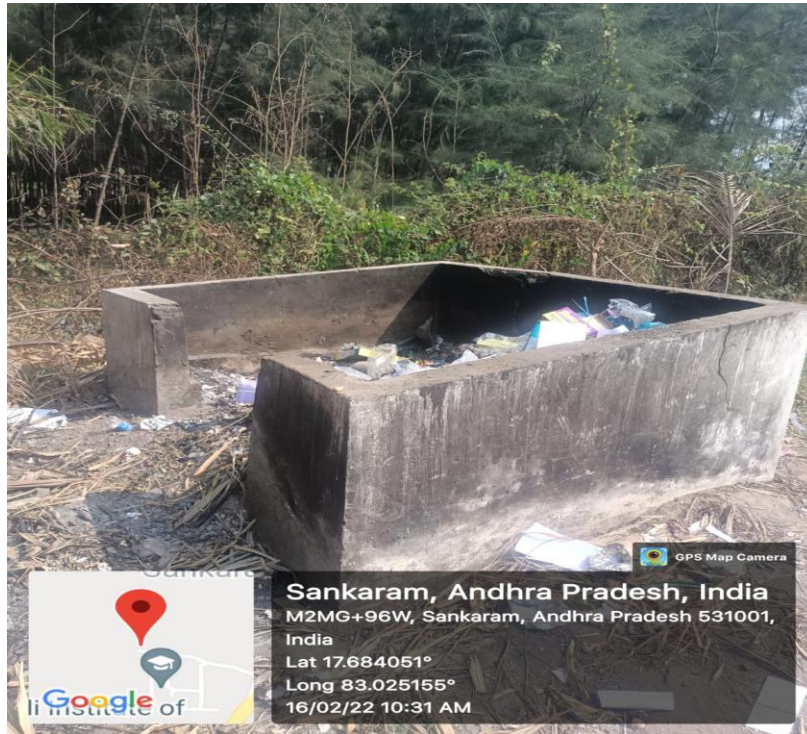
Composting unit Area: 650 Sq.ft Composting Bin Volume:600Cuft
