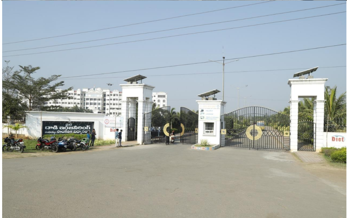
Solar Panels provided at the entrance of the Institution
