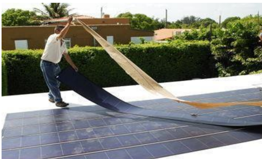
Figure: 1.8 A thin film solar panel composed of non-crystalline silicon deposited on a flexible material.
