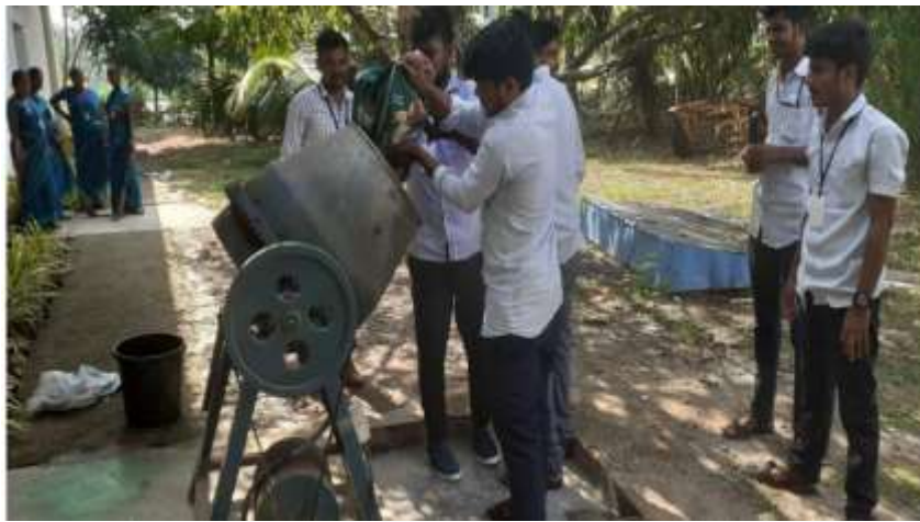
Figure 3.1 Machine Mixing of concrete
