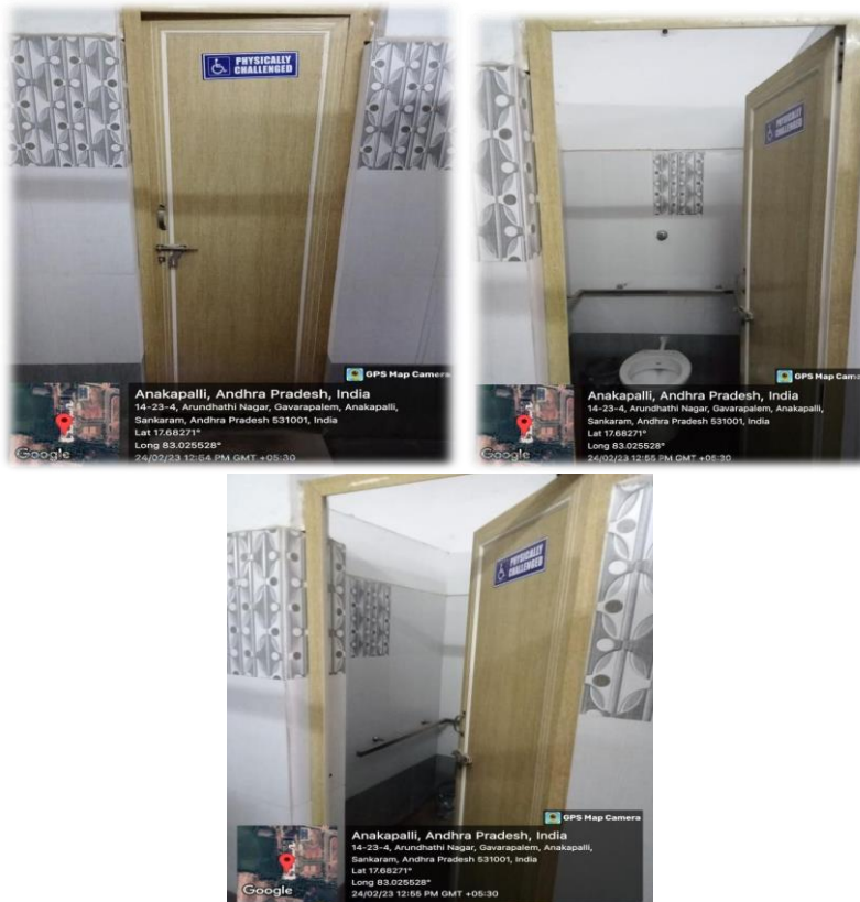
Washrooms for disabled persons
