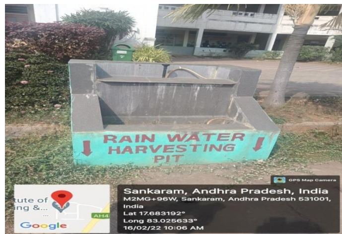
Rain water harvesting pit
