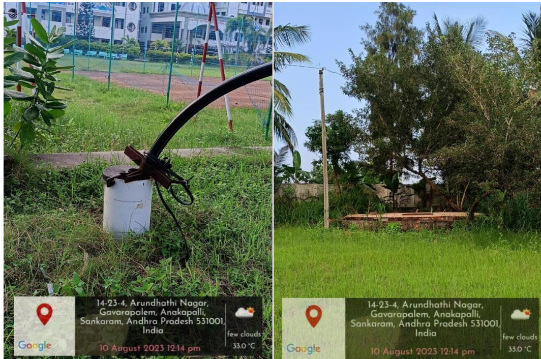
Ground Water Recharge Pit
