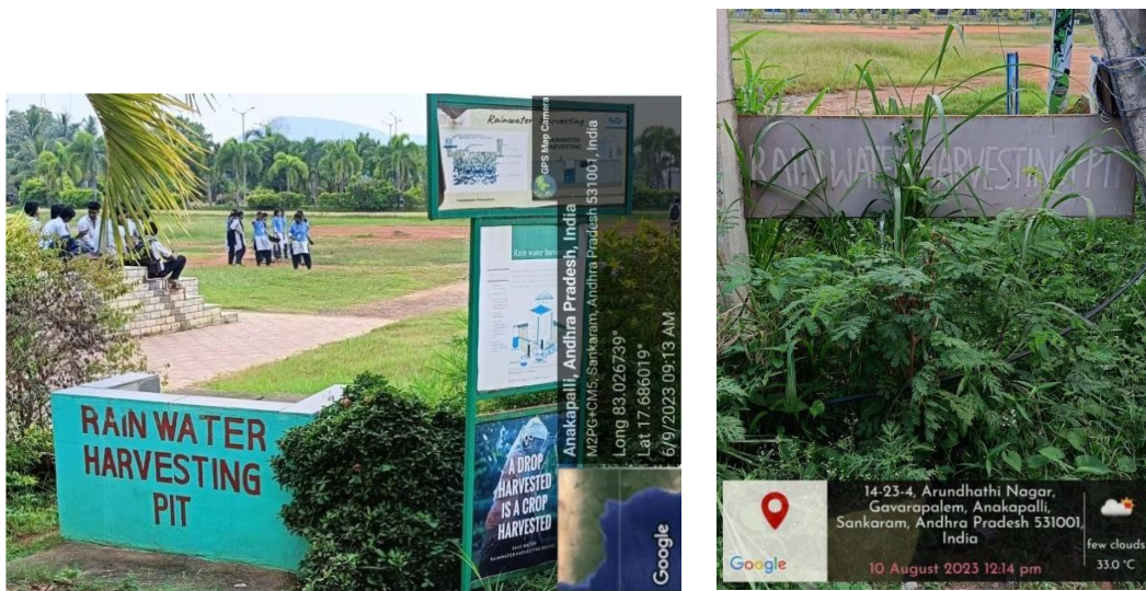
Rain water Harvesting Pit
