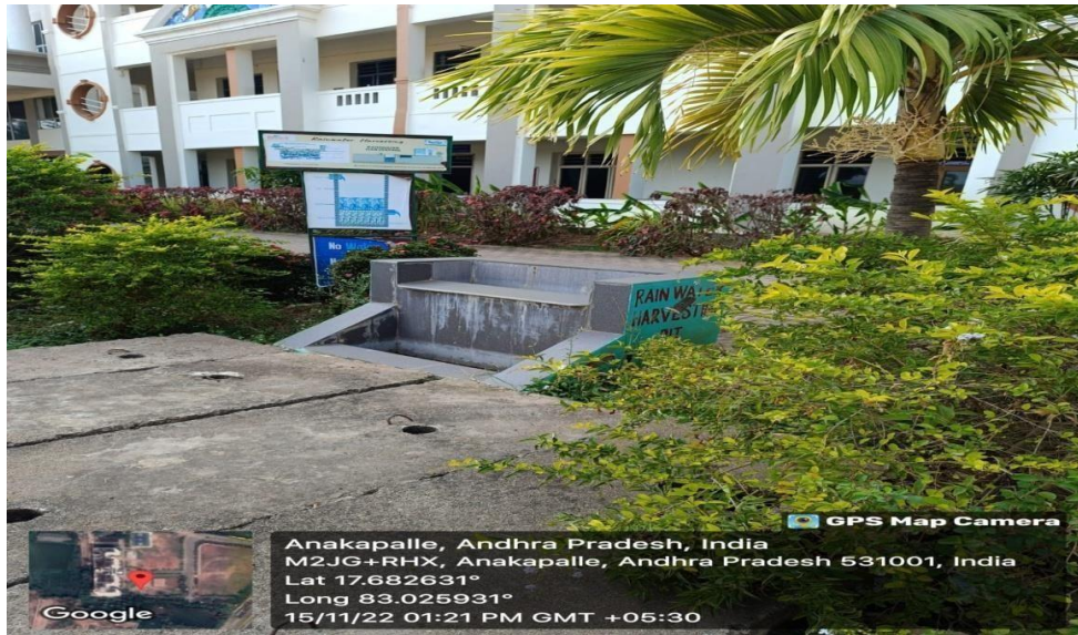
Rain water Harvesting Pit
