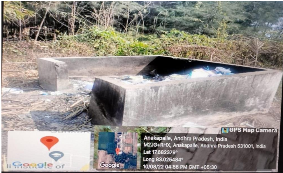
Composting unit Area: 650 Sq. ft Composting unit Volume: 600Cu.ft
