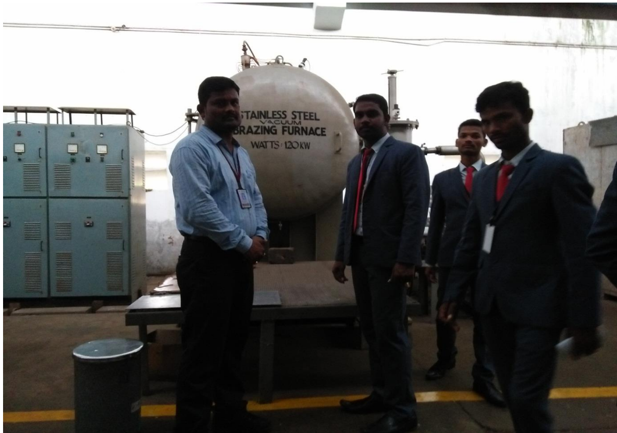
Fig 5:Students at Brazing furnace
